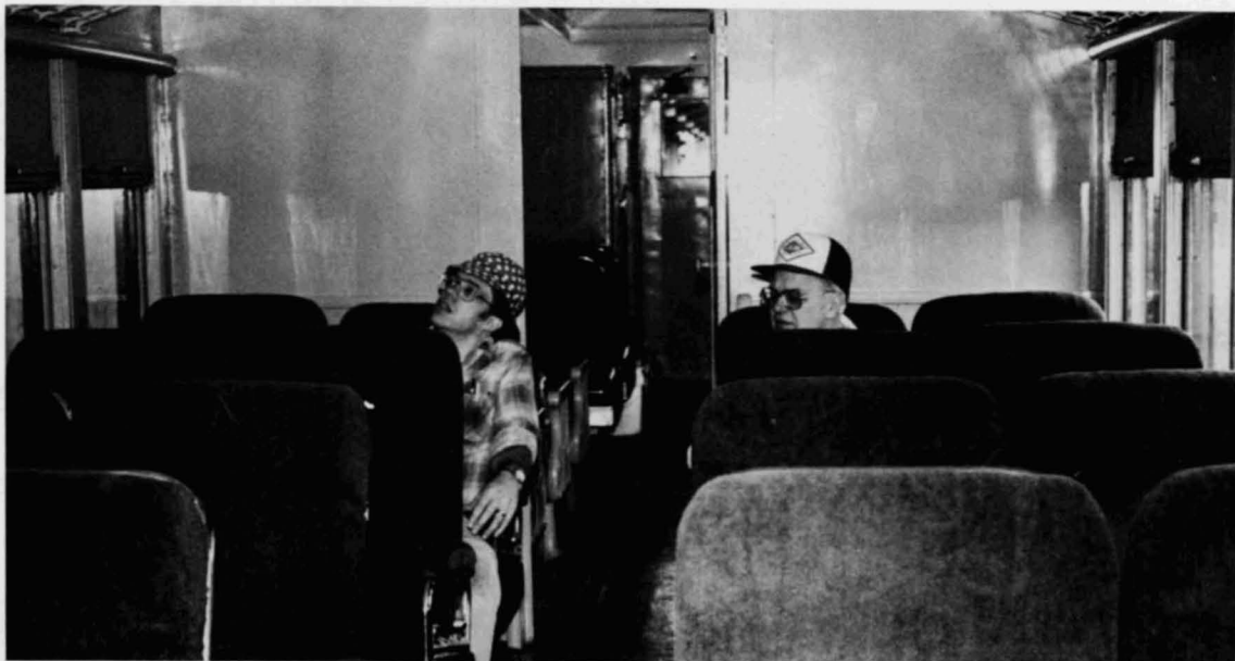
Kurt Haubrich and Bill Mickelsen try out the seats that were just installed in LS&M coach 85.
