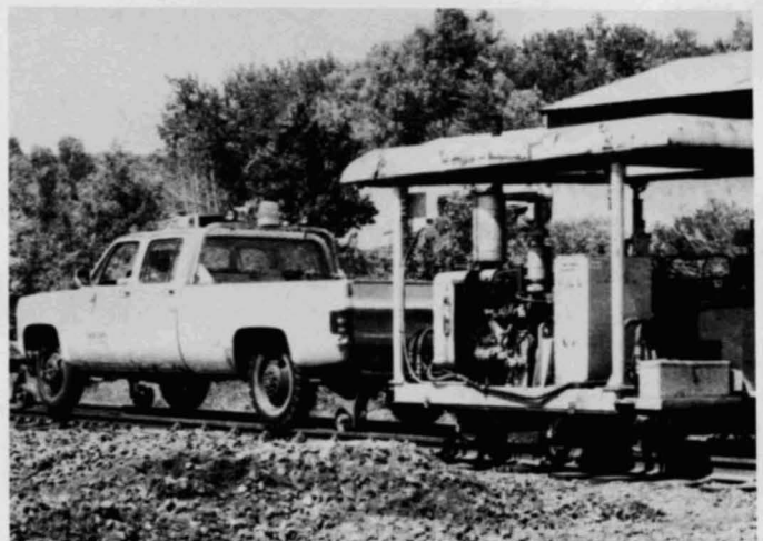
Dick Hanson's high-rail truck, a 1980 GMC from the CNW, pulls the LS&M's newly acquired gang-spiker in preparation for some weekend track work.
