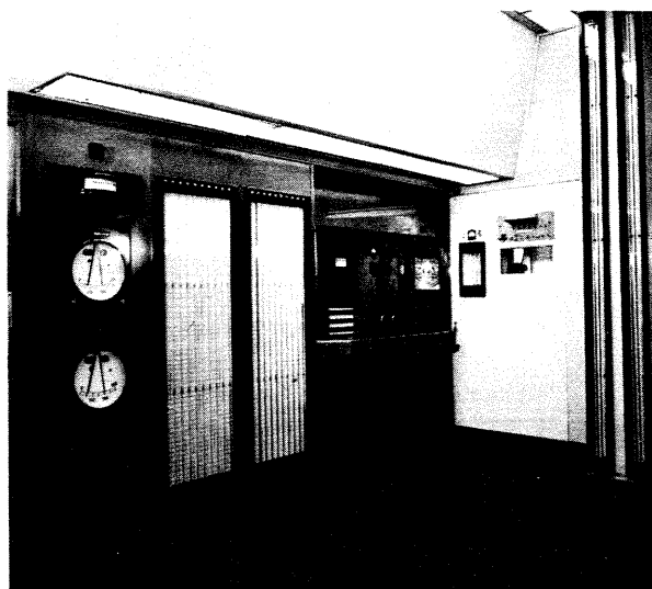
Fig. 23 - Powerplant Test Cell Control Console
